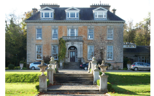
The pond to the front is not original
